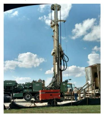
The well bore hole was drilled in decreasing diameters, starting at two feet wide, then down to 18 inches and finally 12 inches wide. The 24" and 18" wide shafts are cased in ductile iron piping to keep the bore hole open. The first 250 feet of the 12" section of the hole is cased in stainless steel.
