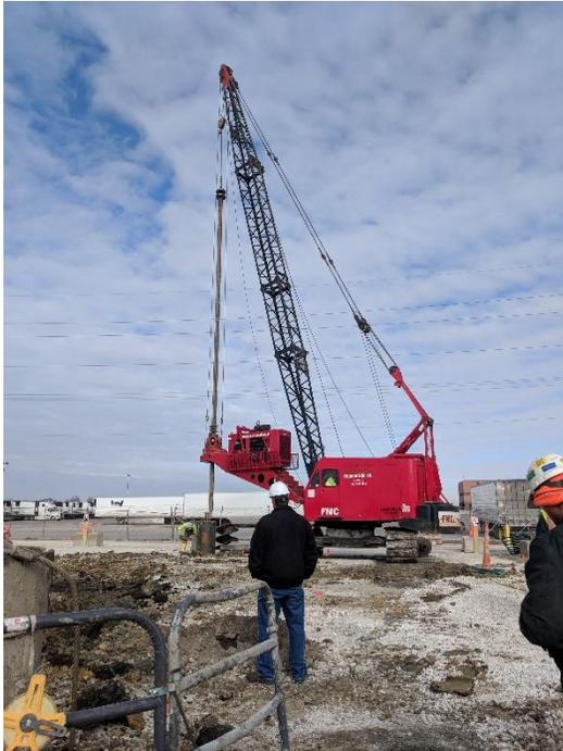
This new building will be 22,000 square feet and will be fire sprinkled throughout. The building will sit on over 100 concrete pilings due to the condition of the ground.
